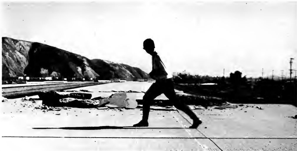
Photo 13. Dislocated roadbed, view southeast along new Freeway 210 (west lane) near Maclay Avenue. Both overthrusting and left-lateral offset occur in line with the San Fernando fault zone.
